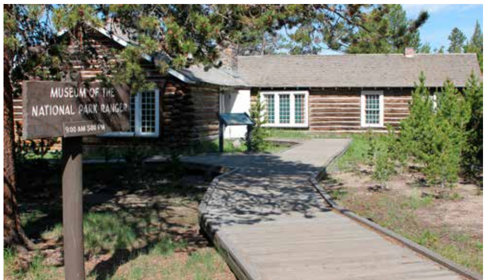
Museum of the National Park Ranger at Norris Campground, taken in 2013. ANPR is pledging to raise funds to help revitalize the museum. Photo: Diane Renkin / NPS
